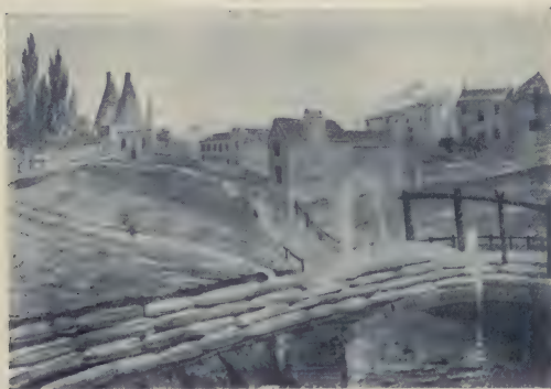
Fig. 42. Wooden water mains crossing the Fleet at Holborn.
